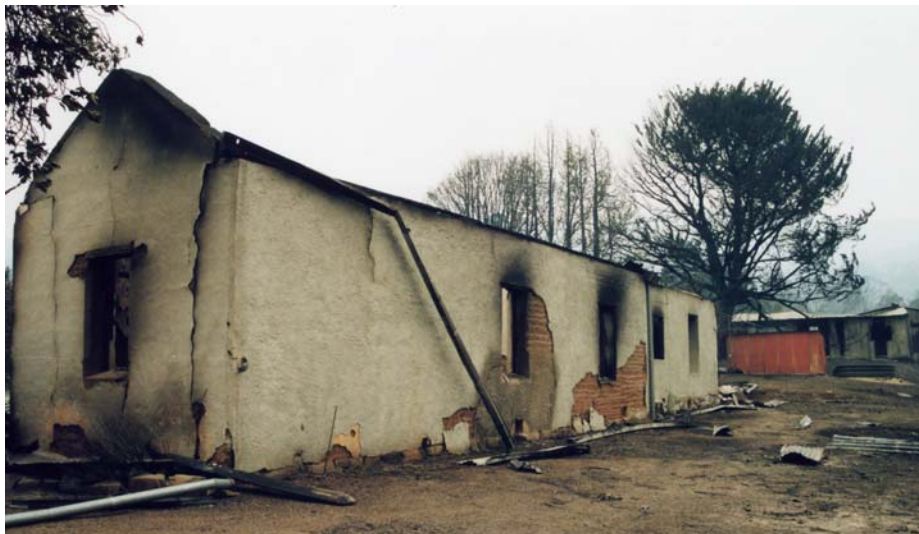
Built from a “pise” (rammed earth) walled construction, the 117 year old “Rock Valley Homestead” had not escaped the firestorm.
