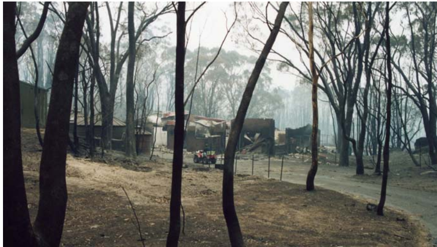
The “Animal House” the day after the Firestorm swept through.
